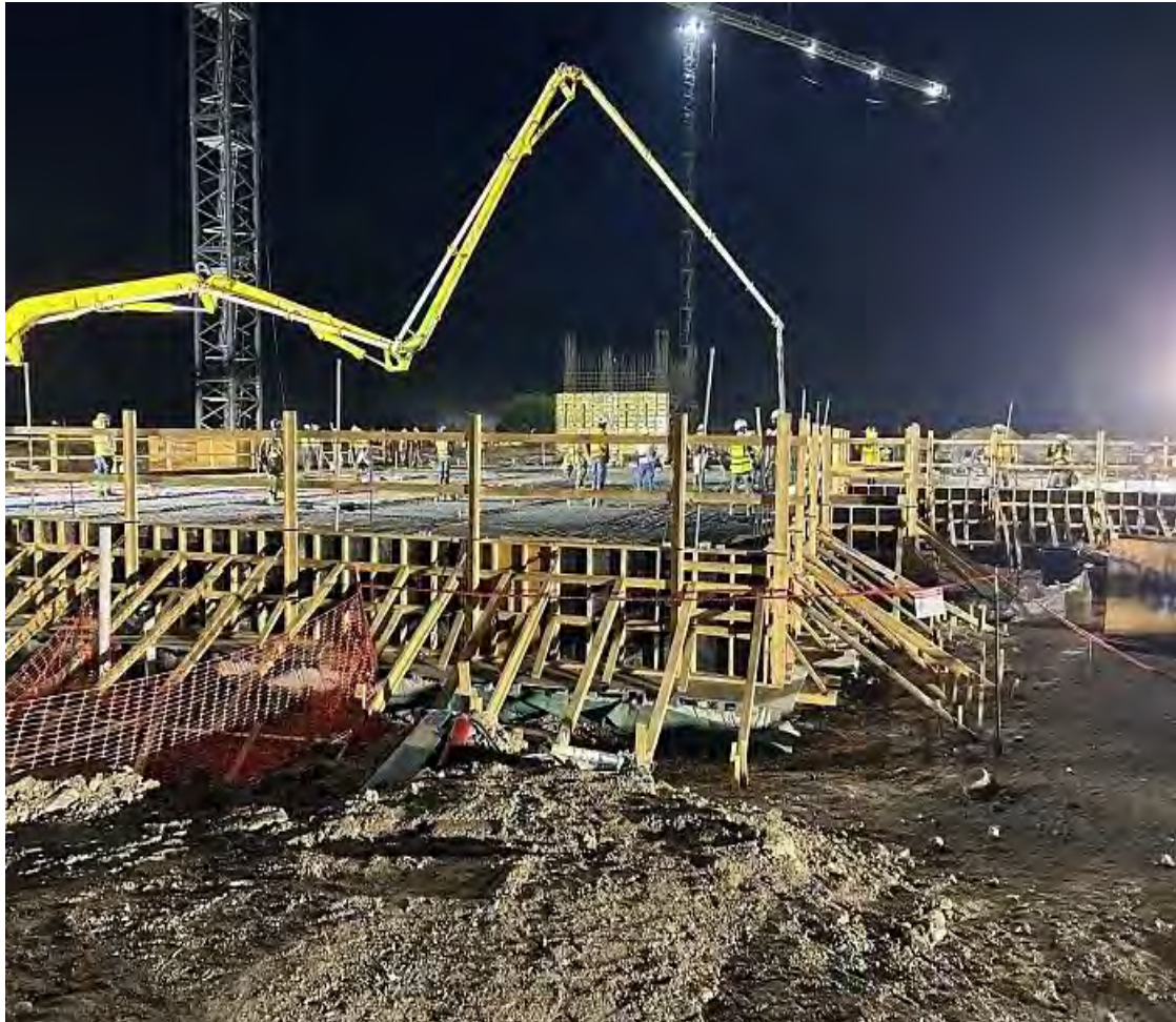
First Suspended Slab Placement
