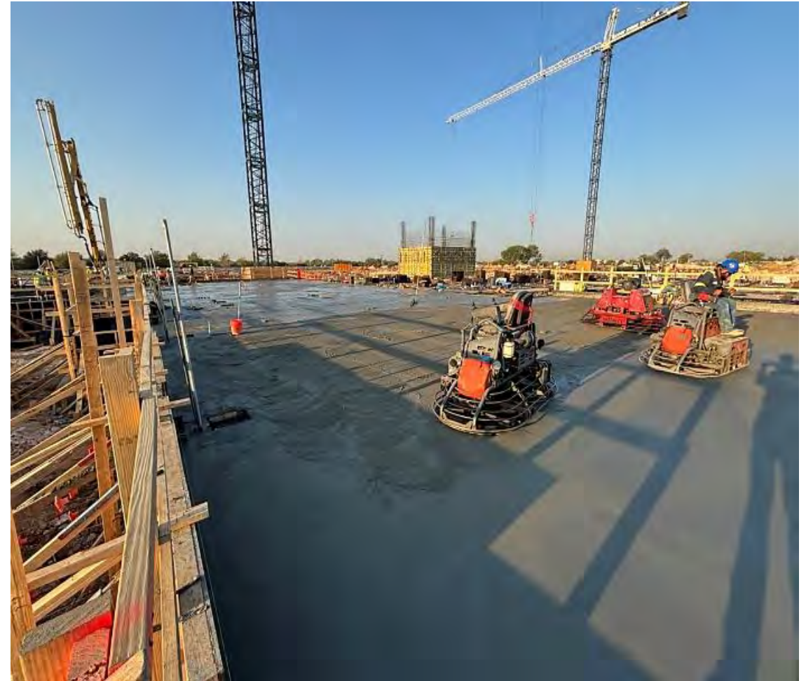
First Suspended Slab Placement
